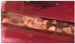
**Recesses or encapsulations:** Areas of recess or encapsulation should be filled very slowly and poured first. Watch for trapped air bubbles in corners, in the detail of objects, etchings, carvings, or crevices. Ease them out by using a tooth pick or other pointed instrument. Do not pour second coat until 3 or 4 hours later.
