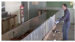
**Aluminum Tape:** If Aluminum tape was used, the tape can be removed when resin has thickened slightly, but still flows. Again, use a brush or foam applicator to assist in uniform coverage and removal of excess resin if needed.
